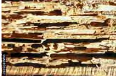
Wood damaged by carpenter ants (R. Werner/IPM Images)
